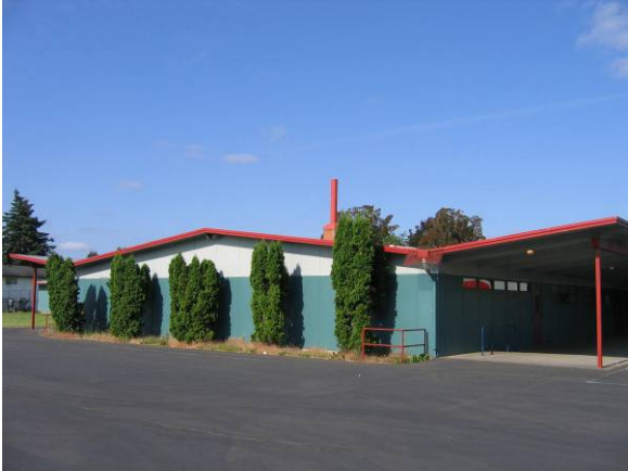
East elevation facing southwest
